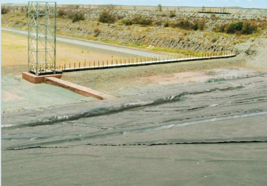
Leg 1 closed with waste rock walls
