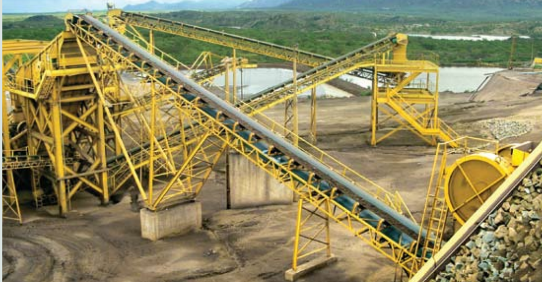
The Mina do Bonito plant
